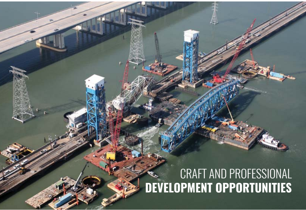
Galveston Texas Railroad Causeway Lift Span Float-In
